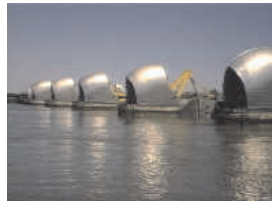
Figure 13: The Thames Barrier.
